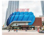
▲ Nansha Wanda Plaza in Guangzhou
